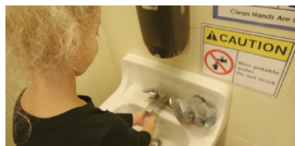
Non-potable water fixture inside Edison restroom
